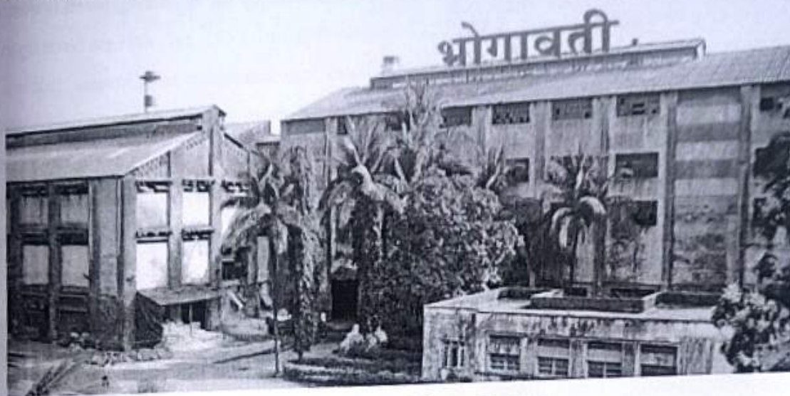
Picture: Bhogawati Sugar Factory
